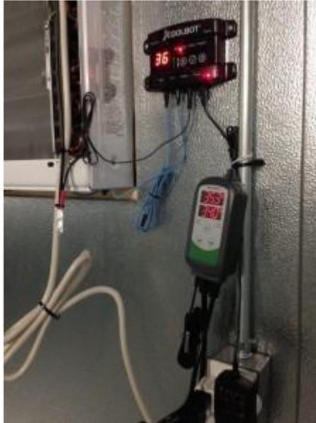
If your INKBIRD Temperature display (the number at the top – labeled PV) is different from the one displaying on the CoolBot, adjust the Temperature
